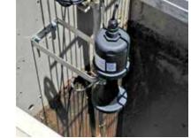
The traditional approach is to use a submersible level sensor. Rags and other heavy paper debris can enter the sewage pipes and tend to wrap around and clog the submersible sensor. This can prevent the sensor from
