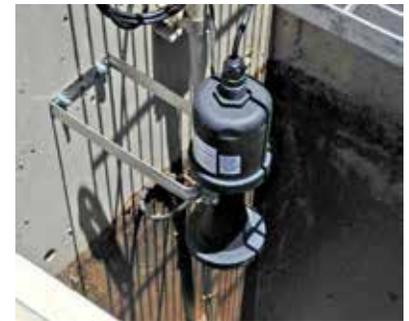
The traditional approach is to use a submersible level sensor. Rags and other heavy paper debris can enter the sewage pipes and tend to wrap around and clog the submersible sensor. This can prevent the sensor from accurately measuring the level and cause an overflow. For this reason, back-up level float switches are usually installed to shut down the pumps if the submersible sensor fails to detect a high level.
